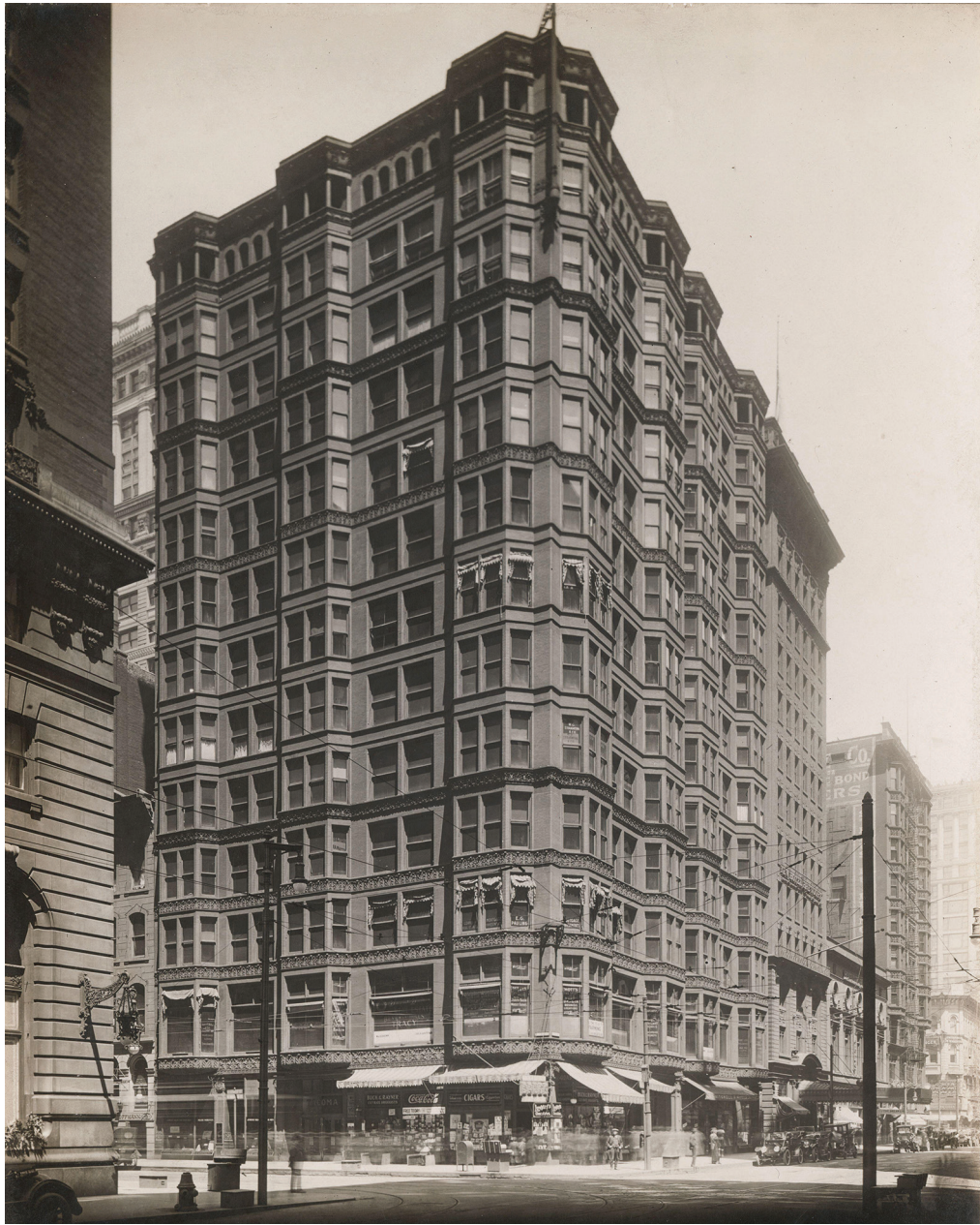
The Tacoma Building was an early skyscraper built in Chicago in 1889.
