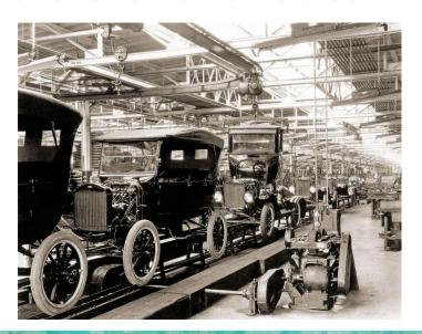
In 1908, Henry Ford introduced the Model T, one of the first vehicles made using Ford's step-by-step manufacturing process.
