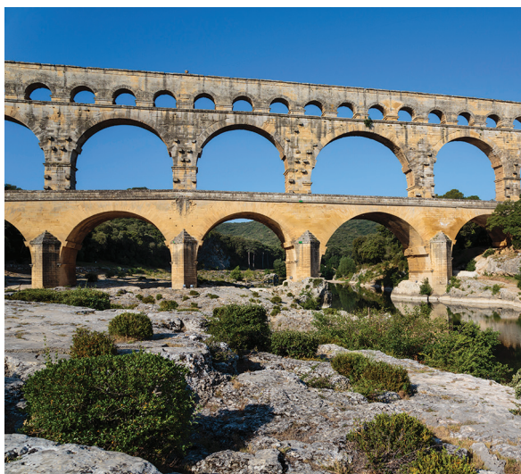
Aqueducts, like this one in modern France, brought clean water to distant parts of the Roman Empire. The arches made the structure very strong.
