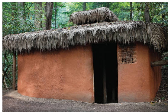
This structure is a replica of the kind of house that some Cherokee people lived in. It has plaster walls and a thatched roof.
