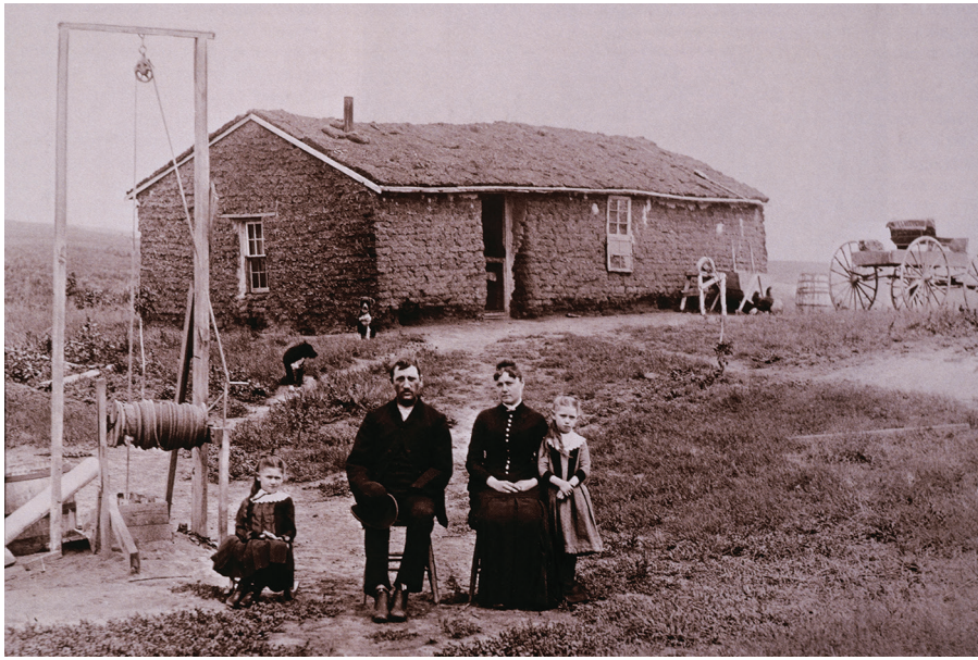
This house was made from sod bricks with a sod roof. There were very few trees or stones available for building houses on the Great Plains.
