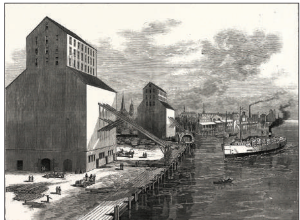
Grain elevators are used to store grain in bulk and then load it onto trains or boats for transport to markets across the country.
