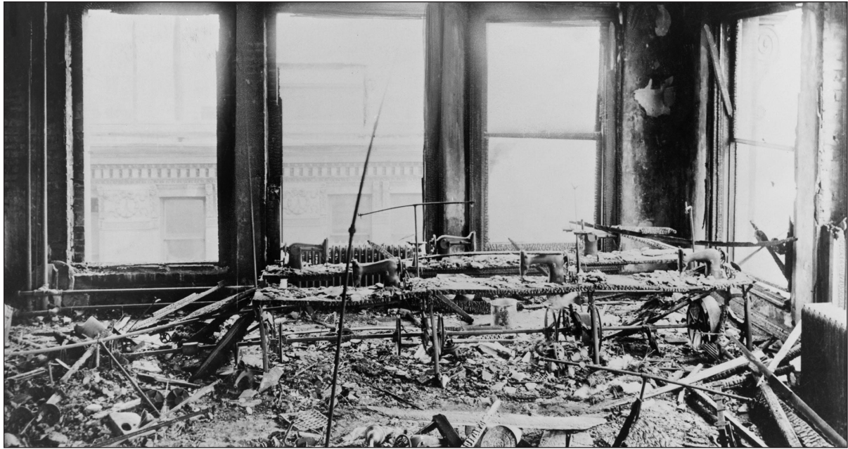
Destruction in one of the workrooms at the Triangle Shirtwaist Factory
