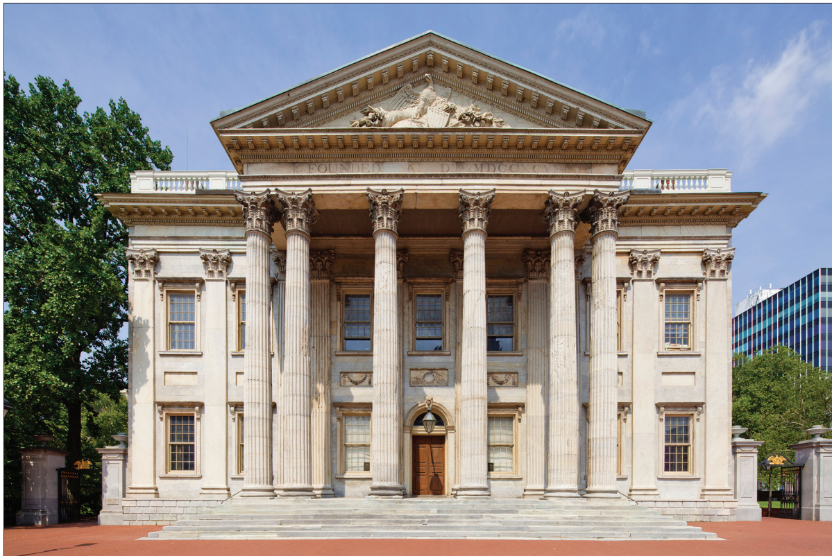
Alexander Hamilton founded the First Bank of the United States, commonly known as the First Bank, in 1791. While no longer a bank, the building still stands today in Philadelphia.
